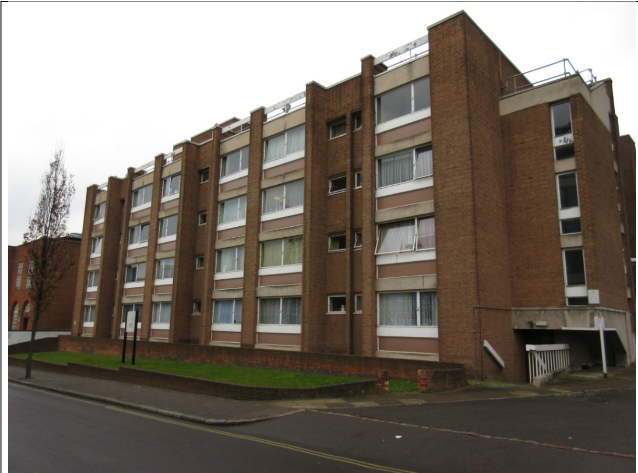
EXISTING LODGE ROAD ELEVATION
